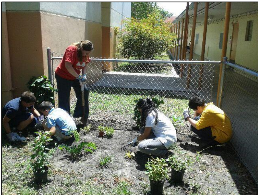
Figure 4. Teacher and 5 th -grade students working together to construct the butterfly garden at North Hialeah Elementary School
